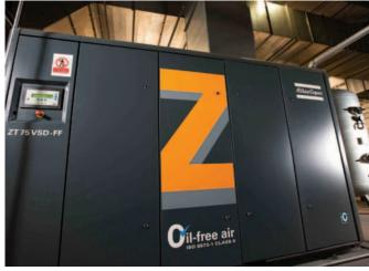
Copco ZT37 fixed speed, oil-free compressors and associated refrigerant dryers with a single air-cooled ZT75VSD FF machine, incorporating the IMD heat-of-compression adsorption dryer – which eliminates moisture before it enters the air net in order to ensure
